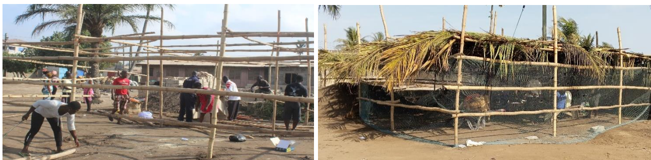
Figure 3: Construction of nursery shed.
